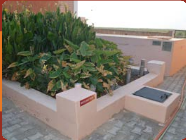
Energy efficient and eco-friendly phyto-remediation STP plant
