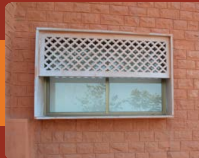
Local Jodhpur stone is used for the facade, Wall thickness is 18 inches to reduce the heat ingress to provide a comfortable temperature inside, naturally.
