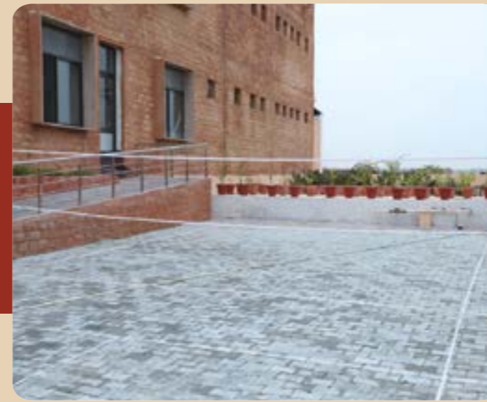
Paver blocks, planters and water body to reduce heat island effect for microclimate.
