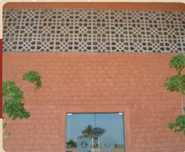
Traditional Jodhpur Jali helps in reducing heat ingress, it allows light and airflow.
