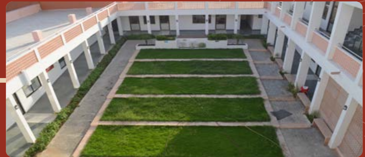
Paver Blocks and planters working as a heat reducer
