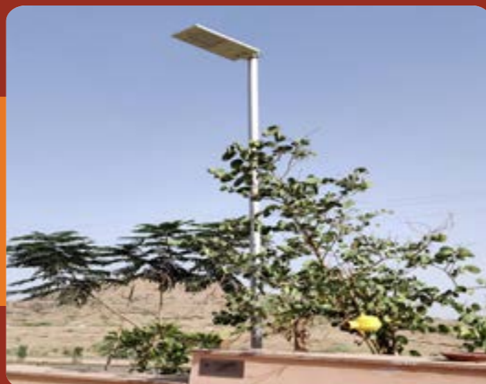
Solar Street light facing downwards ensures the building is not only reducing its carbon footprints but also taking care of its eco-system by minimizing light pollution for enhancing the nocturnal life of animals
