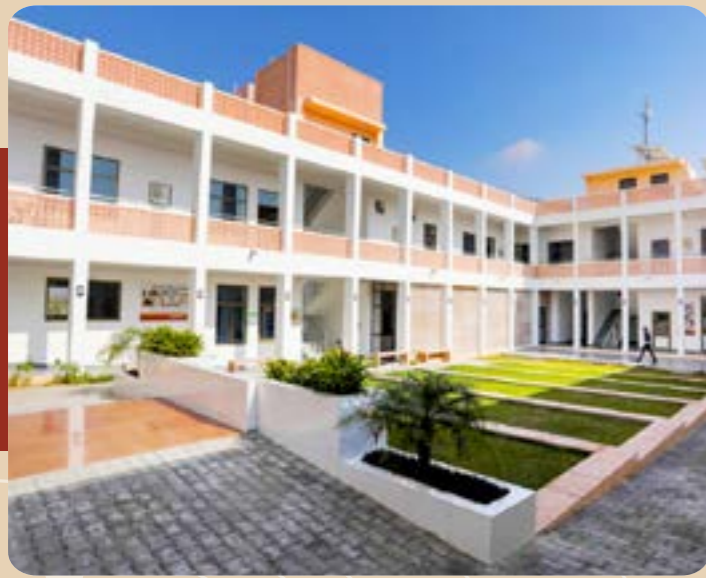
The central part of the building is open to the sky and lined with open verandah allowing sufficient light visibility, this also provide excellent natural ventilation of the entire premises.
