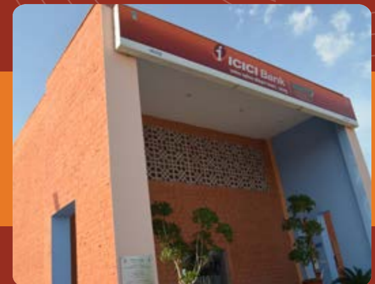
This double-height Foyer enhances the beauty, channelize wind flow from south-west direction into the courtyard, hot air will exit by virtue of stack effect.
