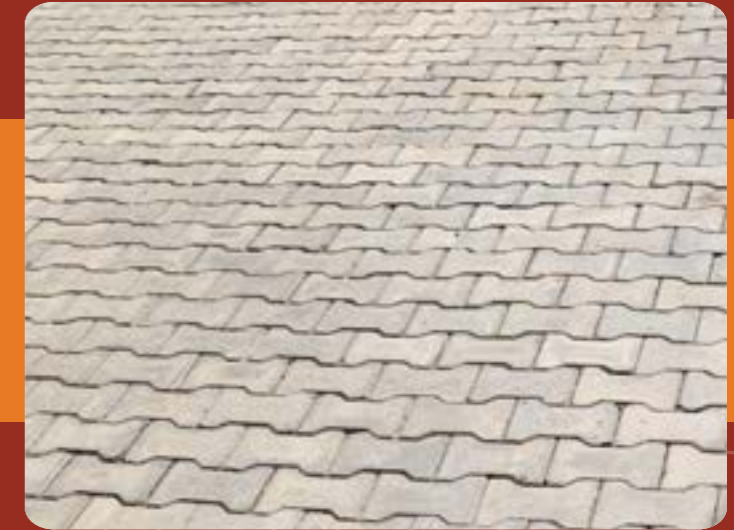
Interlocking Paver Blocks, allows rainwater infiltrate into the ground
