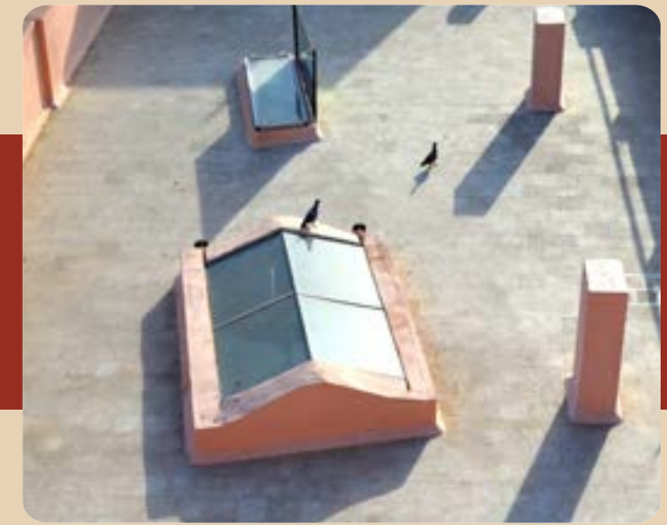
Tiles with a very high solar reflective index (SRI) used on for roofing to minimize solar heat gain.
