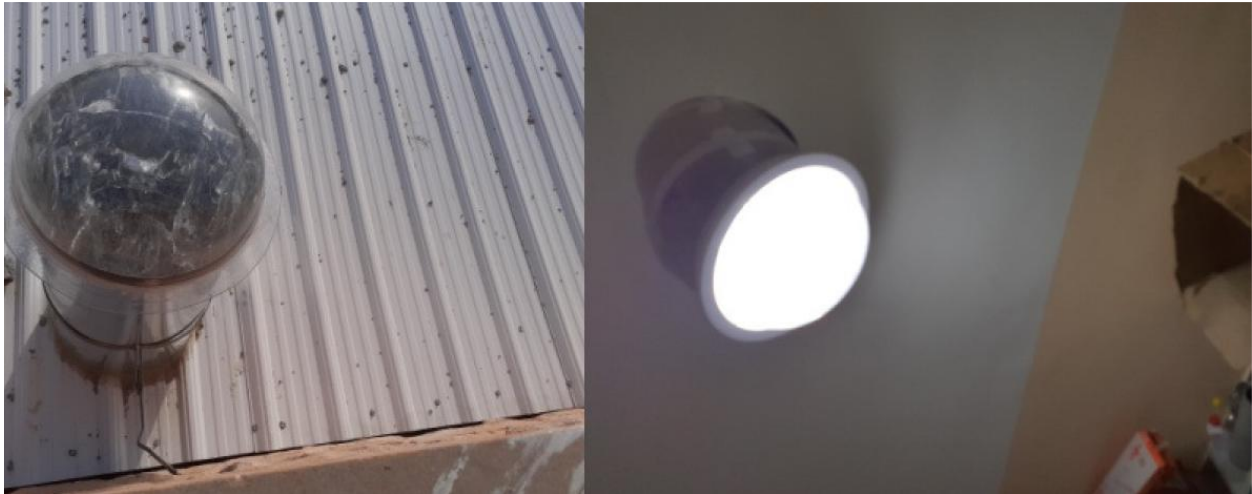
Fig 17: Light pipe used in medical room
