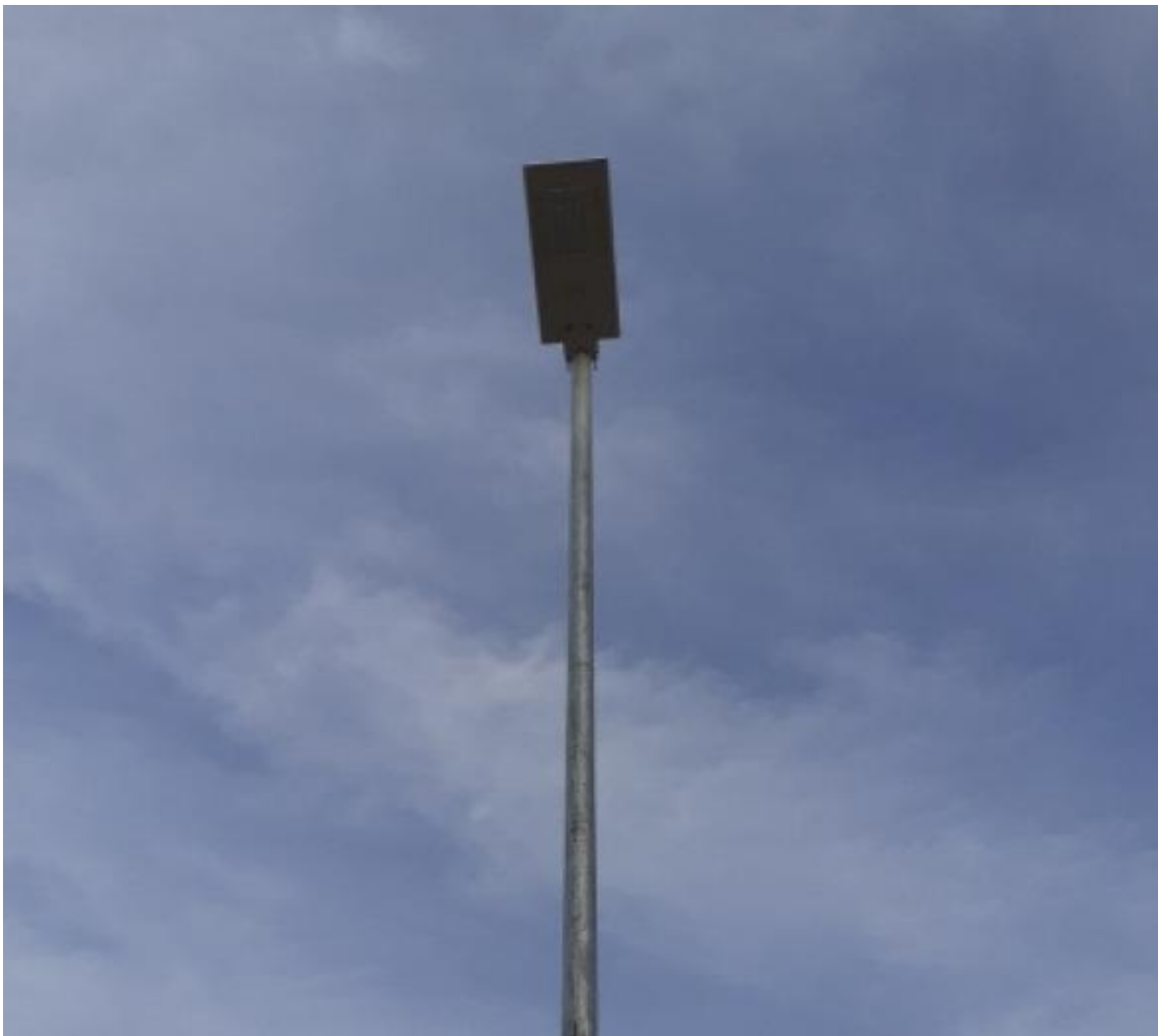
Fig 7: Solar photovoltaic street down-lighter
