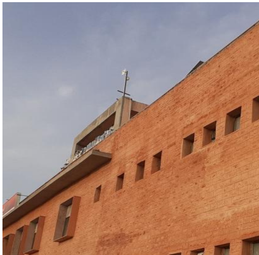
Fig 11: East facade of building
