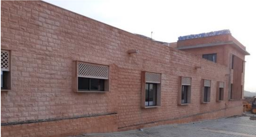
Fig. 12: Shading cum ventilation on the South side of the building
