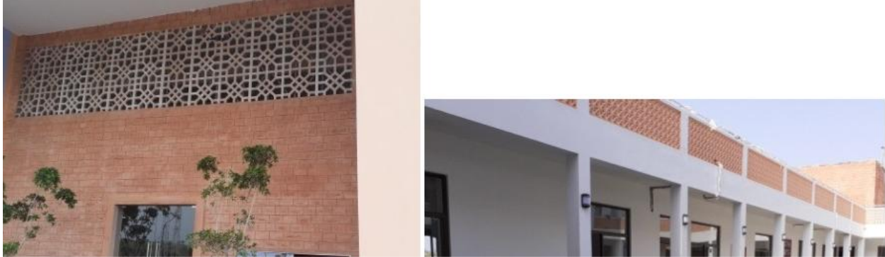
Fig 10: Natural ventilation provisions
