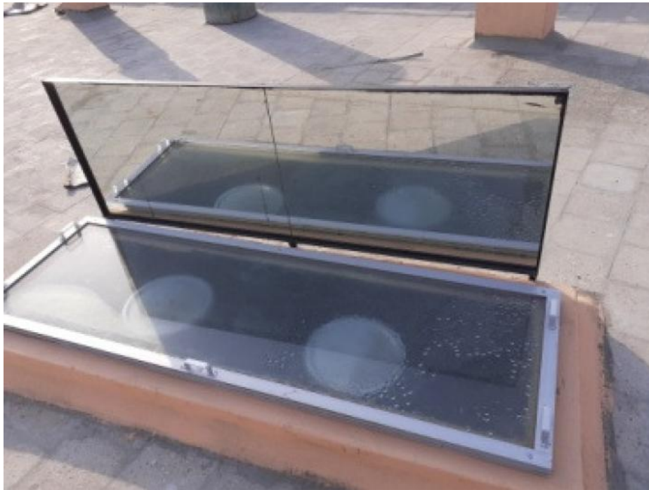
Fig 13: Built in solar cooker on roof
