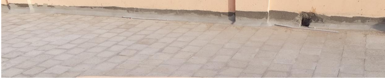
Fig 8: Cool roof tiles on entire roof
